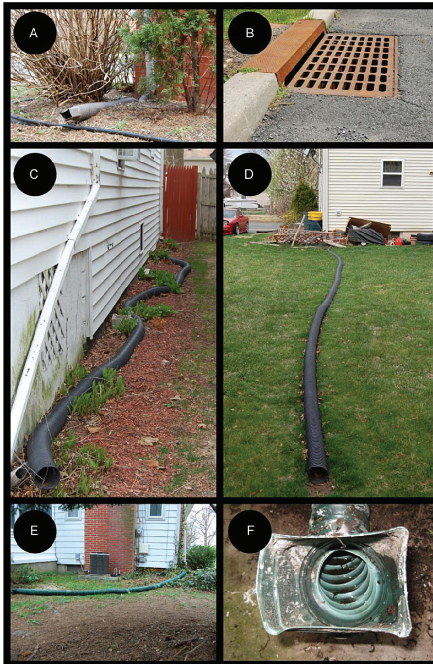
Figure 1. Examples of corrugated extension spouts (CES) within residential backyards in the New Jersey, USA. All CES within this figure were holding water and contained immature Aedes albopictus . (A) Brown CES with a square opening and incorrect pitch. (B) Example of a catch basin located at the curb. (C) and (D) Elongated black CES displaying excessive length (>10 m) and flat pitch that allows water accumulation in the folds. (E) Elongated green CES with flat pitch. (F) View of the inside of a CES viewed from the side originally attached to the rain gutter downspout. The small pockets of water in the folds are a cryptic habitat for immature A. albopictus .
